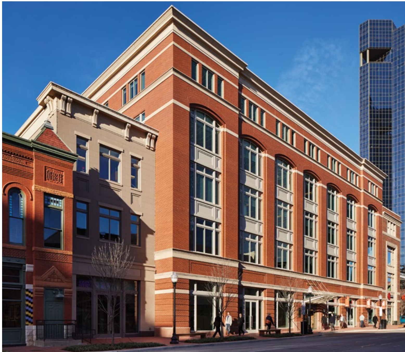
Above: Commerce Street facade. The primary volume of the Commerce Building is framed by two components articulated as separate structures. The north bay is known as the Acorn Building; the cast-stone border around its windows features oak leaves and acorns. The south bay, composed in buff stucco, serves as a link to the historic Land Title Building.
