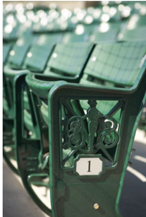
Above: Spectator seating. The seating bowl was renovated with refurbished seats from the Orioles' home field of Camden Yards.
