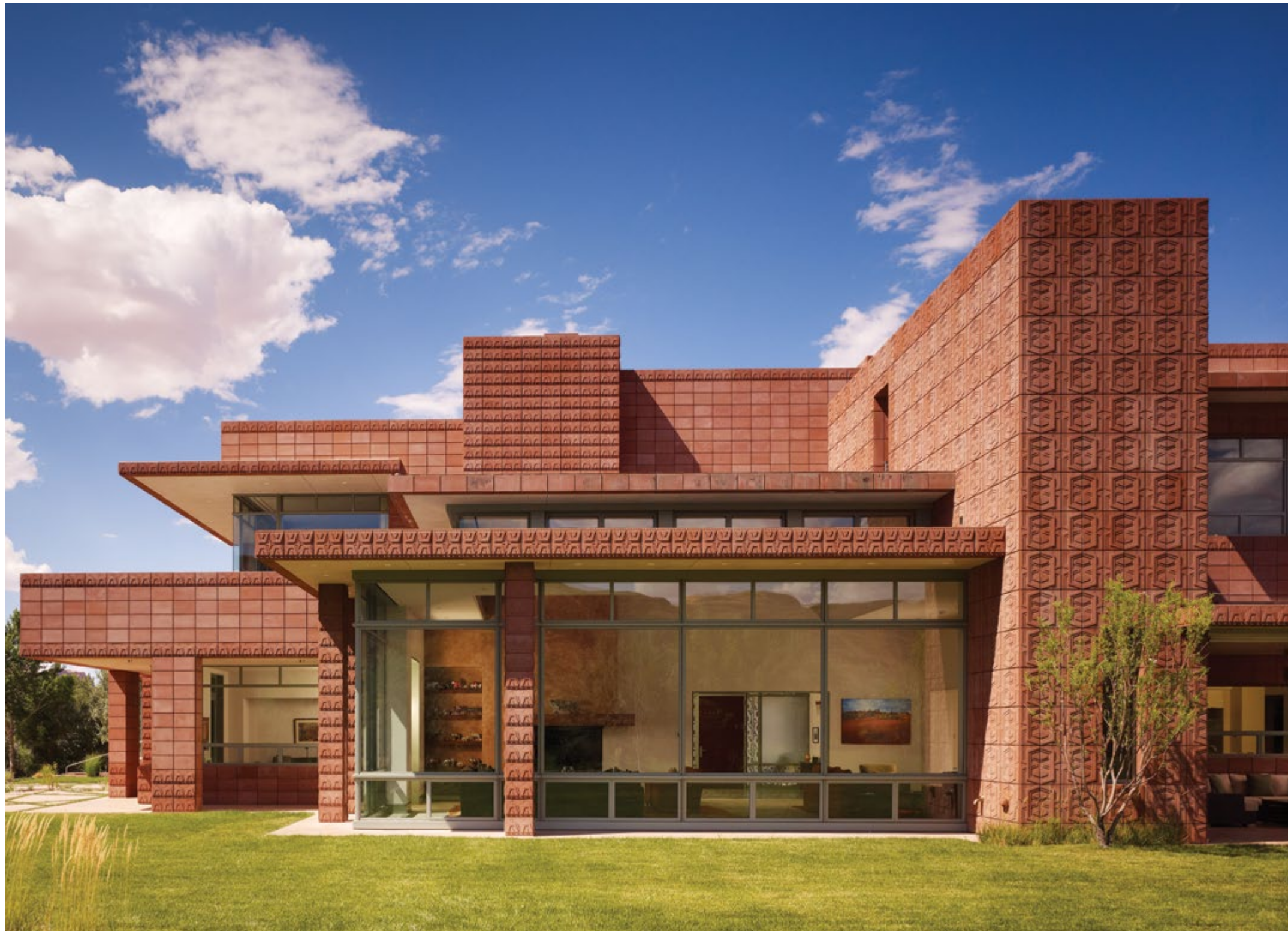
Above: Southwest corner, main house. Deep roof overhangs and terraces shade the large expanses of glass of the south-facing interior spaces. The custom cast-stone block of the building walls was based on a stylized geometric pattern inspired by the landscape.
