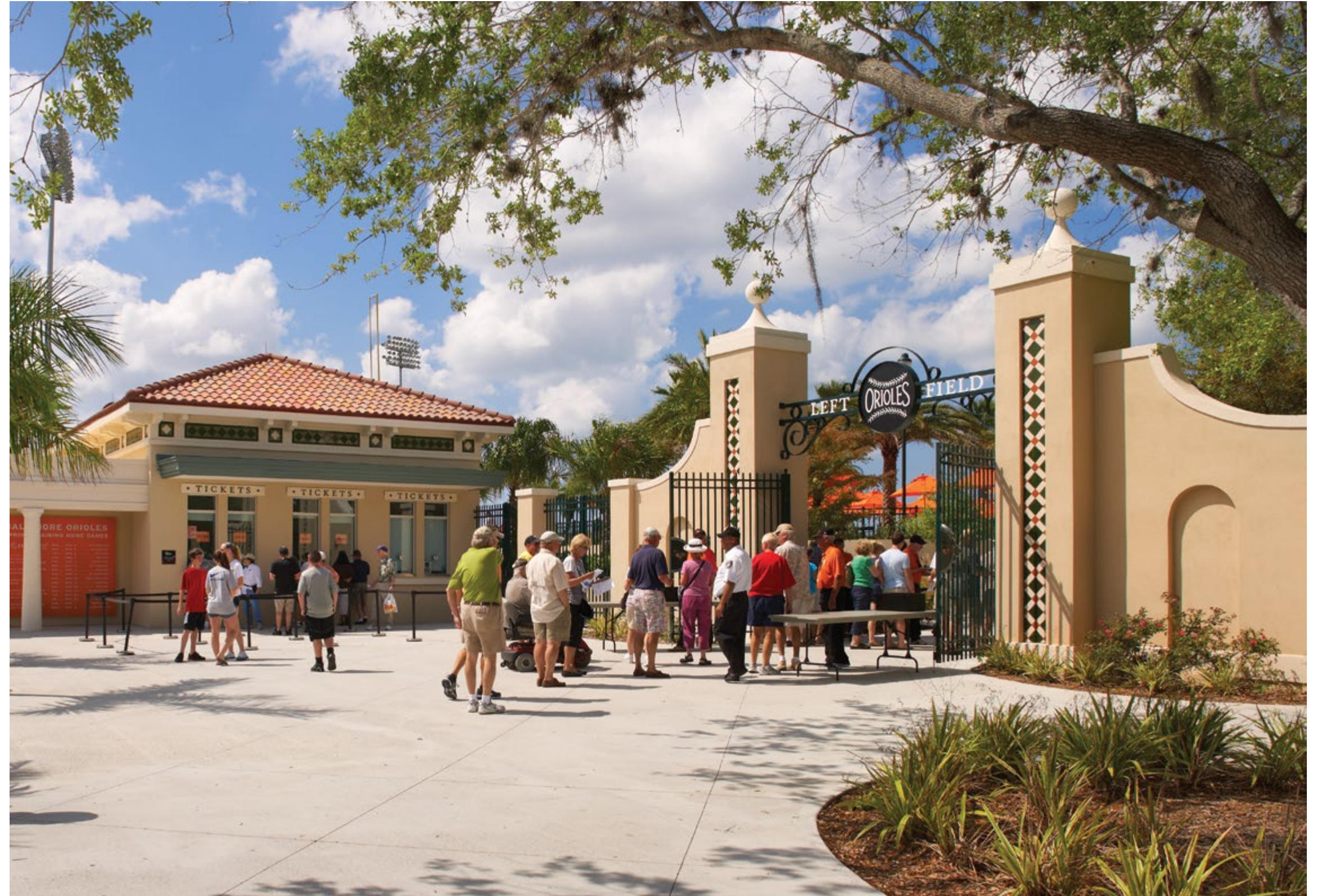
Above: Left field entrance. A new ticket and concession building and a formal entry gate share the materials and details of the ballpark. Concrete roof tiles in a custom red blend unify the various structures of Ed Smith Stadium and complete the link to Sarasota's "Florida Picturesque" past.
