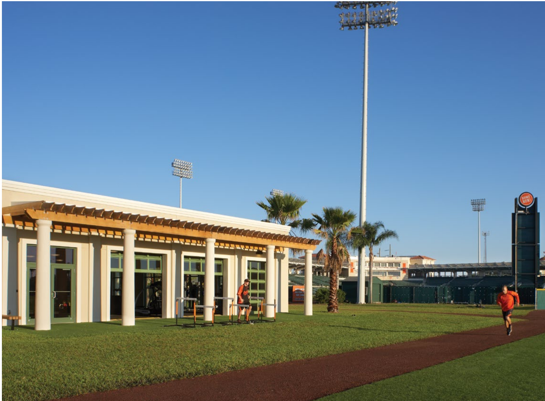
Above: View from southeast. A trellis of cypress and stucco-clad columns shades the glass garage-style doors between the weight room/agility area and the practice fields.
