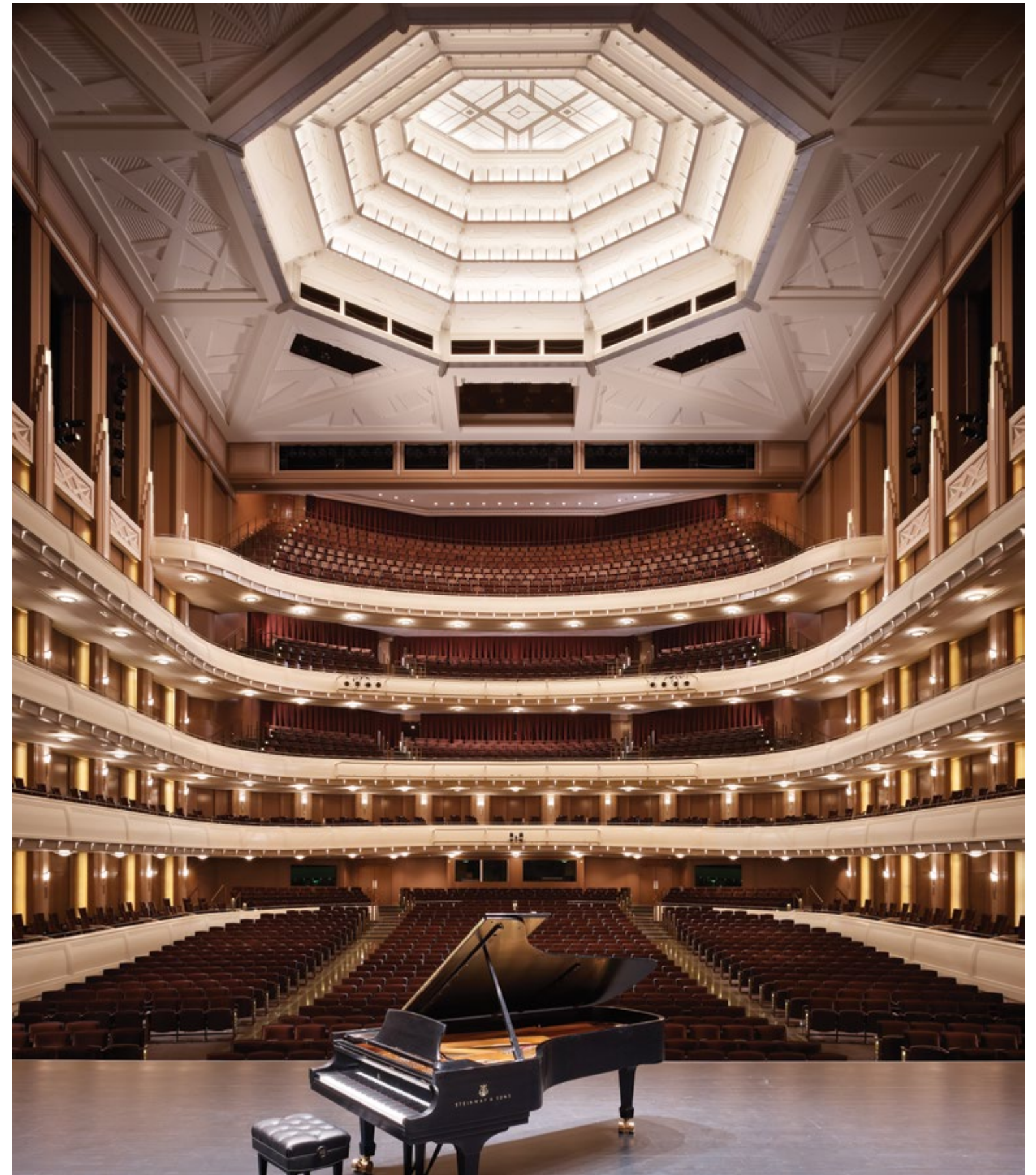
Opposite: Ceiling of concert hall. Crowning the auditorium is a series of stepped glass and aluminum light covers and a horizontal laylight. Although it was constructed as a series of ceiling layers, this element was conceived as a singular chandelier that unifies the space yet does not conflict with sight lines from the balcony, a common problem with traditional chandeliers.
