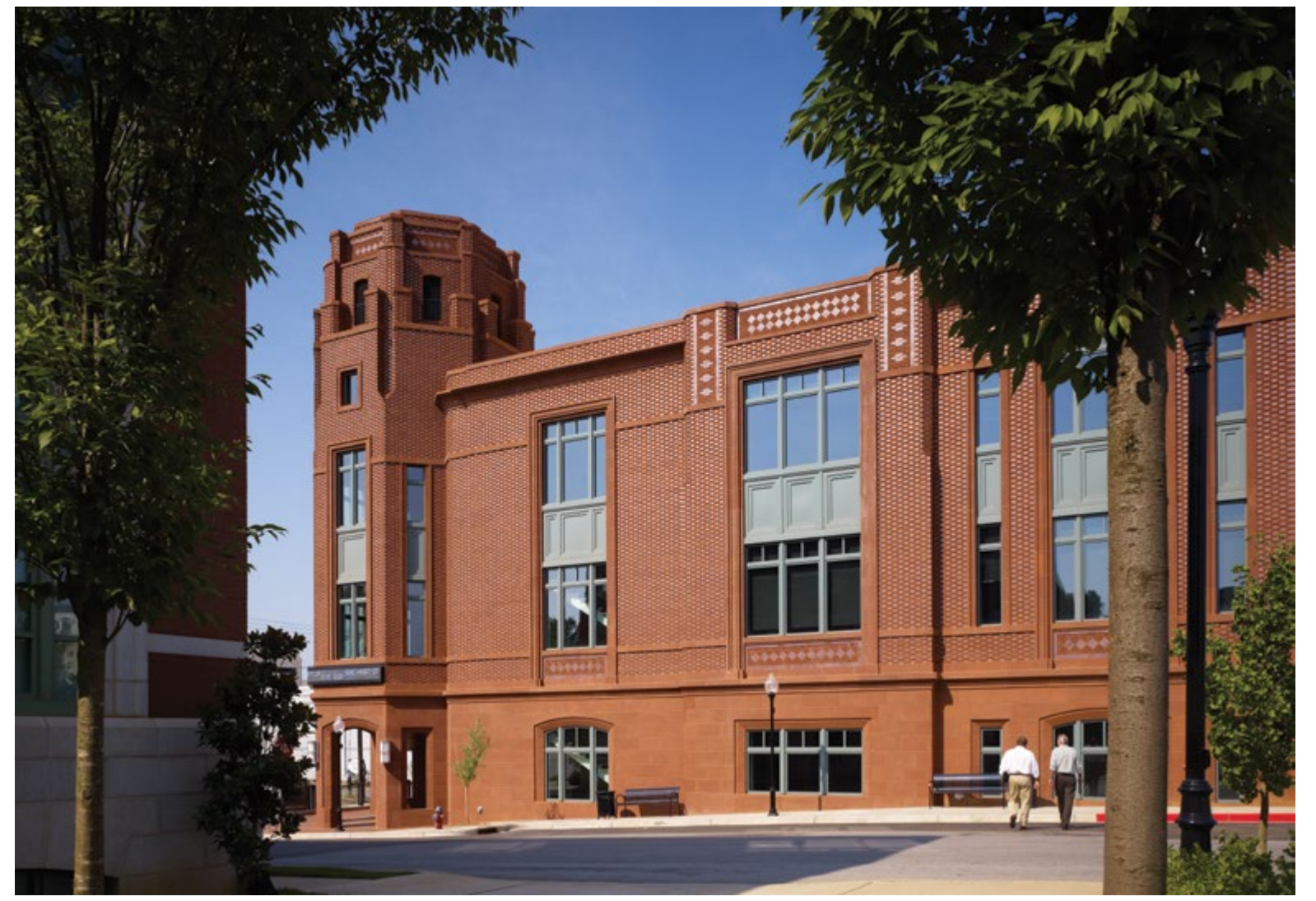
Opposite: Detail of one bay, St. John Street facade. Cast-stone trim, Flemish bond brick patterns, and metal-framed windows create depth and texture. Large expanses of glass flood the 60,000-square-foot building with natural light.
