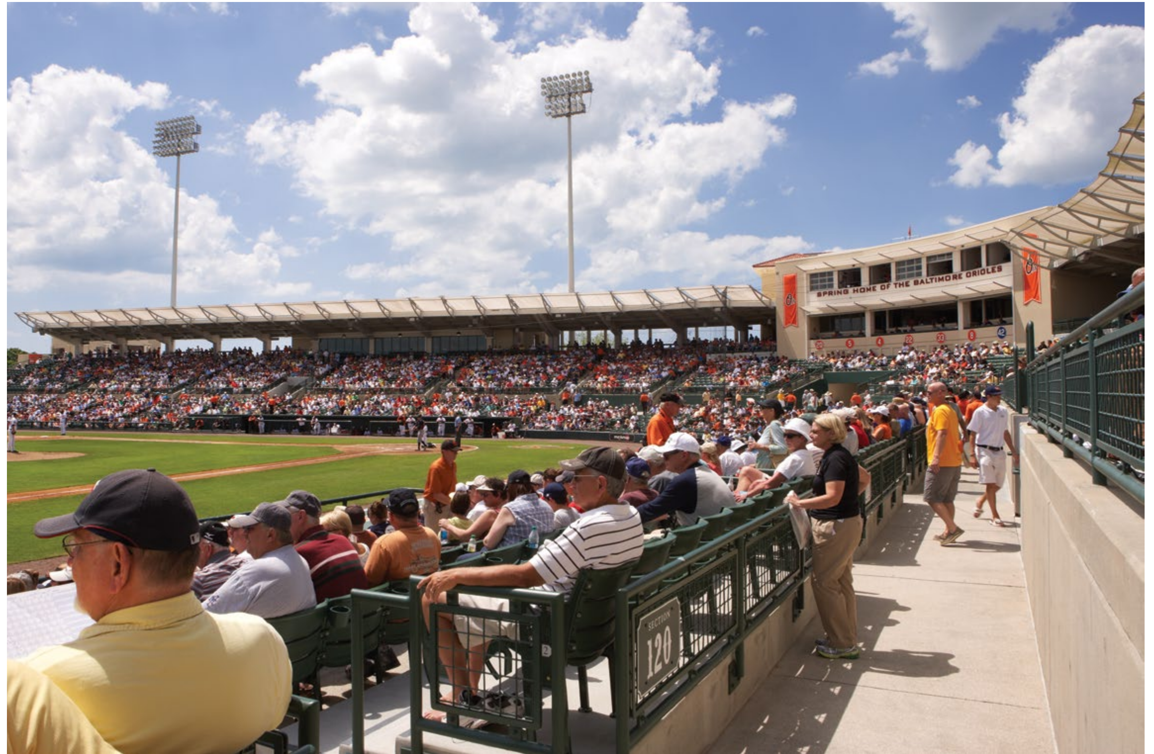
Above: View along third base line. Two new rows of seating along the cross-aisle increased the number of seats close to the field. A fabric and metal canopy attached to the existing metal and concrete roof greatly expands the number of shaded seats.
