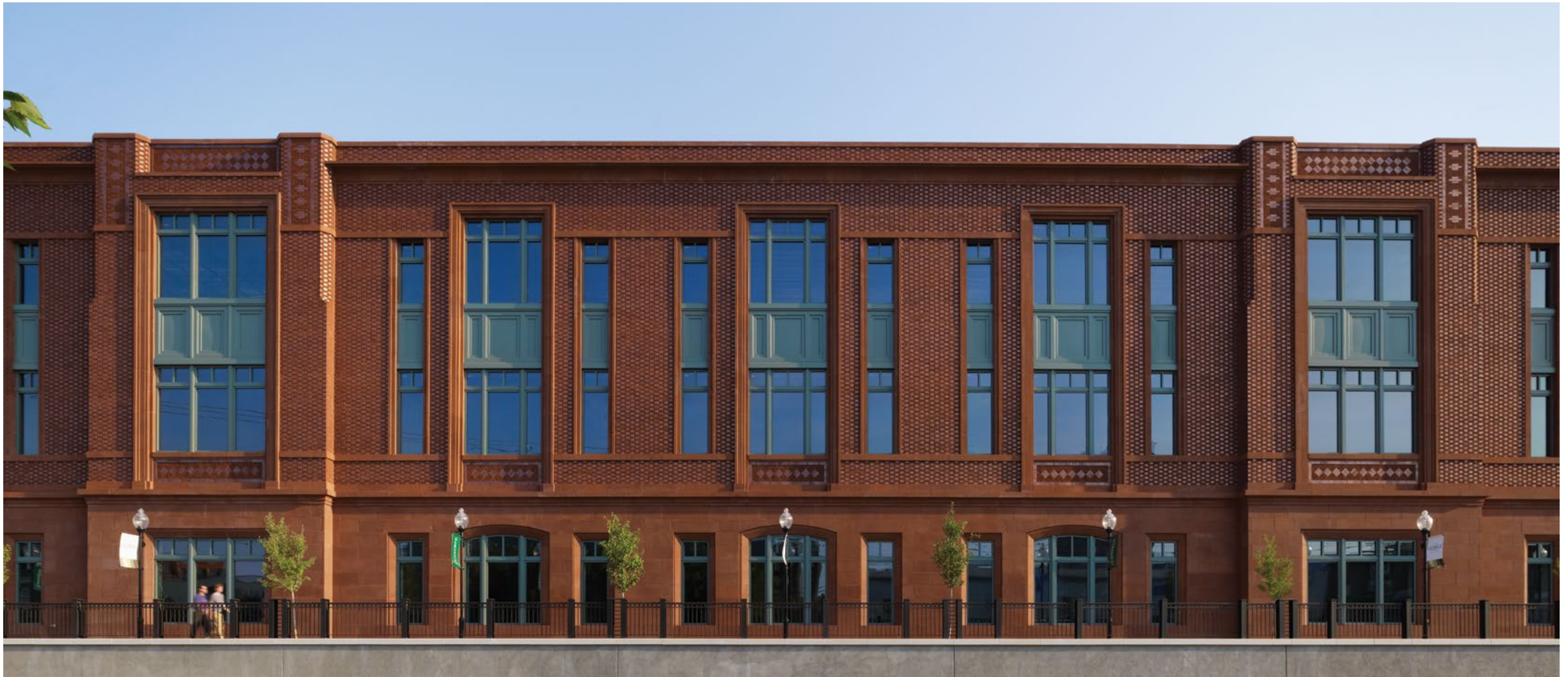
Above: St. John Street facade. The rhythm of windows, trees, lampposts, and railings is dictated by the classroom module within the building. The sidewalk is raised to create a level plinth; the plinth separates first-floor classrooms from the adjacent traffic.
