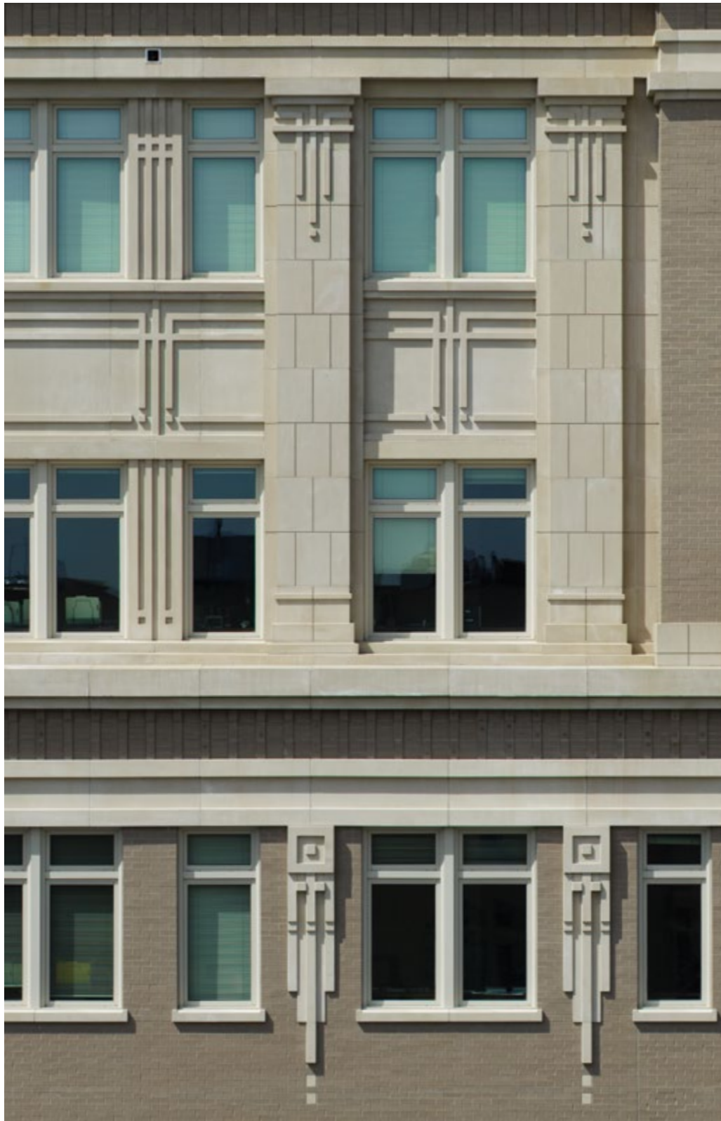
Above: Detail of attic stories. A cast-stone colonnade highlights the top of the building with detailed pilasters and panels. Cast-stone brackets supporting each pilaster introduce Secessionist-inspired detailing that weaves down through the body of the building. Above the colonnade, the top floor steps back to form terraces.
