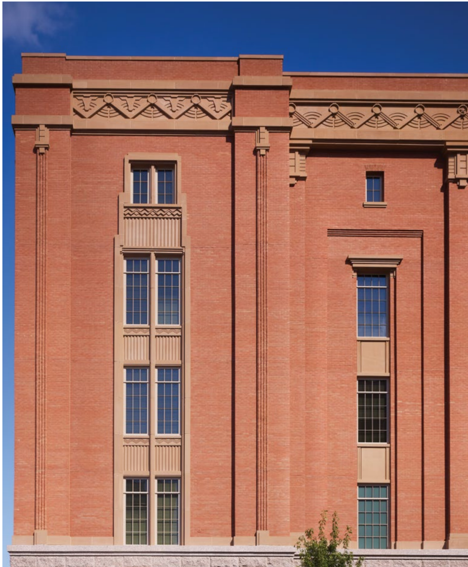
Above: View from south, end tower detail. The composition draws its inspiration from the rich “Cowtown Deco” heritage of Fort Worth, with traditional brickwork detailing and cast-stone decorative spandrels and frieze.
