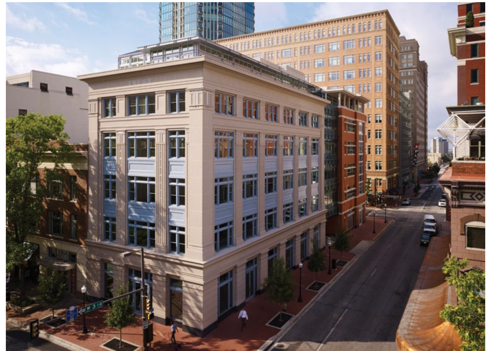
Opposite: View from north, Third Street facade. The bridgelike metal facade spans a ramp for an existing underground parking garage, while the taut brick planes that turn the corner from Third Street to Throckmorton Street conjure early-twentieth-century Dutch architecture.
