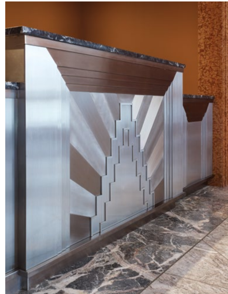
Above: Bar front in main lobby. Patterns based on the sun's rays and the step motif are incorporated throughout the building. Changes in the finish of the stainless steel (polished, satin, angel hair) create the design on the bar's panels.
